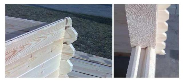
The wall-boards must be placed so that the ends interlock. Now screw the first row of wall-boards into the bearers. All the following rows of placed wall-boards should interlock not only at the ends, but along their length as well. Please screw each new row of wall-boards into the former row to ensure a solid structure. Here is an actual plan of this summerhouse:
